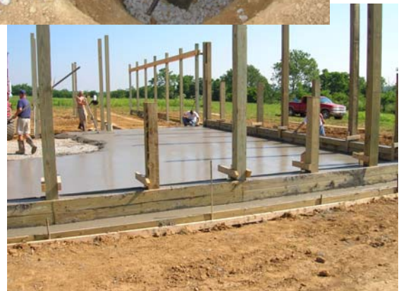
Quality Control Construction Inspections as Required by NRCS
