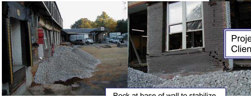
Rock at base of wall to stabilize
