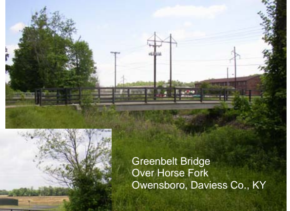
Greenbelt Bridge Owensboro, Daviess Co., KY Photo Taken from Hwy 60 Bypass
